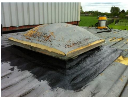
LEAKING TRANSITIONS
