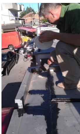
SEAL LEAKING SEAMS
