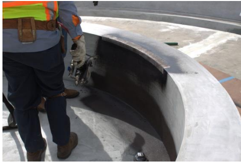
PRE-COAT LAYER OF 1-COMPONENT
