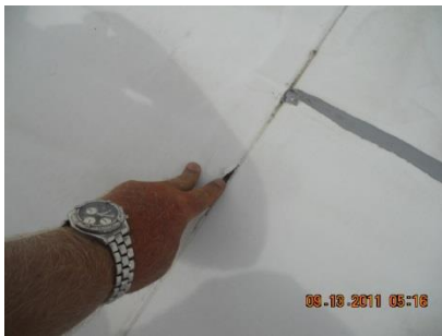
REPAIR LOOSE SEAMS
