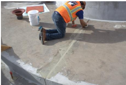
FILL GAPS, VOIDS, OR CRACKS
